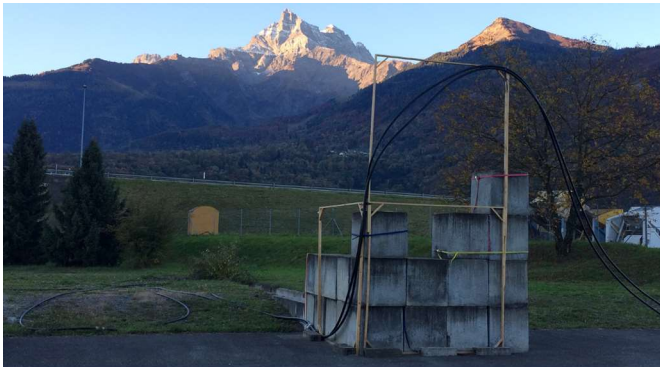
Figure 12. Test trajectory in Bex with ducts in bends in orthogonal planes
