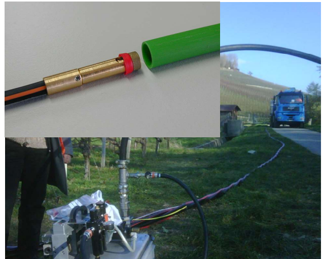
Figure 7. Blowing out with “sonic head”. First prove.
